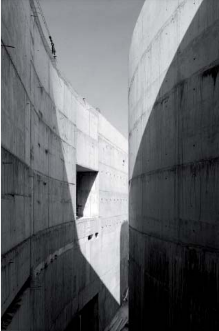
View of the building's passage under construction Photo: Lluís Casals
